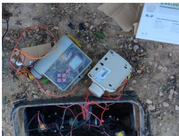
Main road right next to football field (replace broken RainBird programmer with a new Solem)
