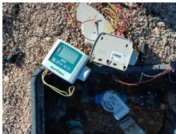
Final roundabout C/ Bahamas (broken RainBird programmer change for used Solem)
