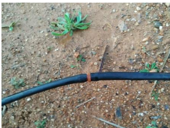
Back garden Phase 6 (5 breaks in PE Ø16-links)
