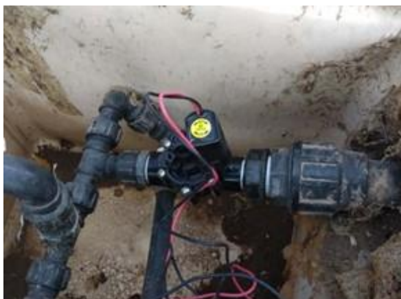
Phase 6 groundabout (change programmer Solem 4 stations and 1 solenoid valve 1")
