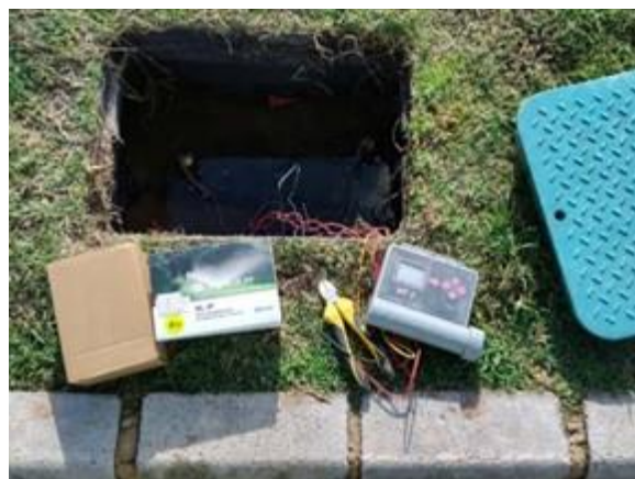
Phase 1 groundabout (change programmer Solem 4 stations)
