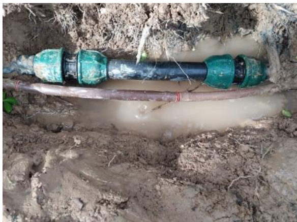
Main road right, maintenance height (0,5 ml PE Ø32 and 2 links)
