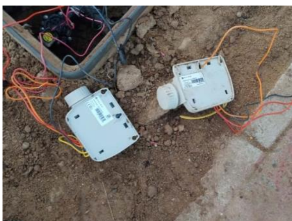
Main right-hand road in front of hotel (change of broken Solem programmer with new Solem)
