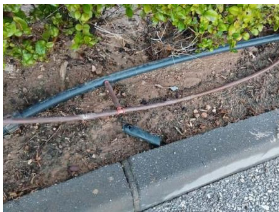
EUM roundabout (2 ml PE Ø16 y 2 links)
