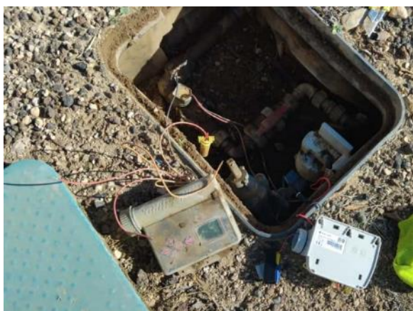
Main road right next to Golf School (replace broken RainBird programmer with a new Solem)
