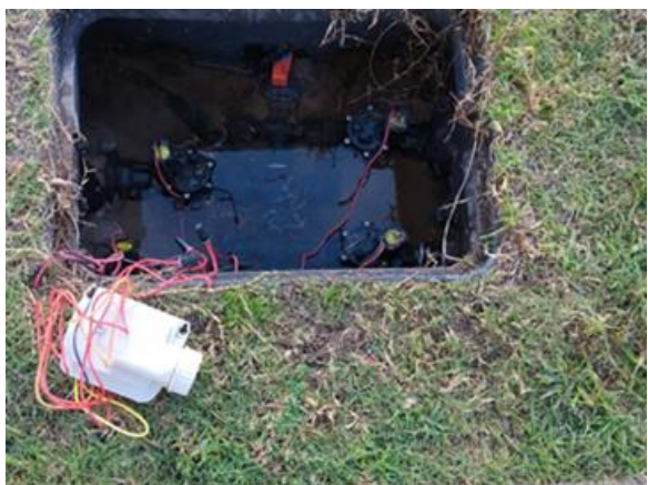
Phase 1 groundabout (change programmer Solem 4 stations)
