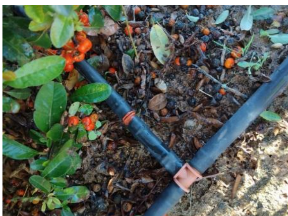
Main road median (4 breaks in PE Ø16-links)
