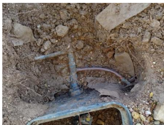
Roundabout C/ Bahamas (0.5 ml PE Ø16 and 1 link)
