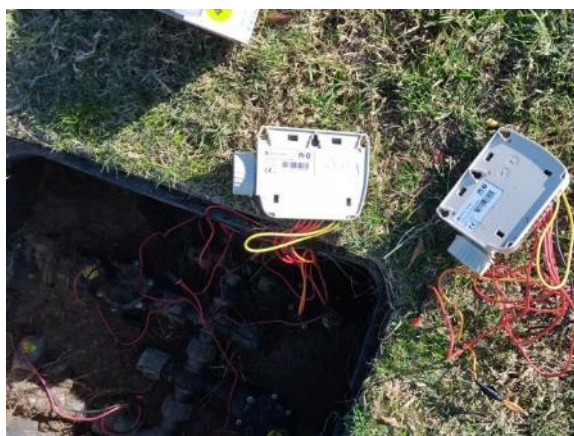
Phase 6 Roundabout (new Solem programmer not working; change with another) NOT ACCOUNTING
