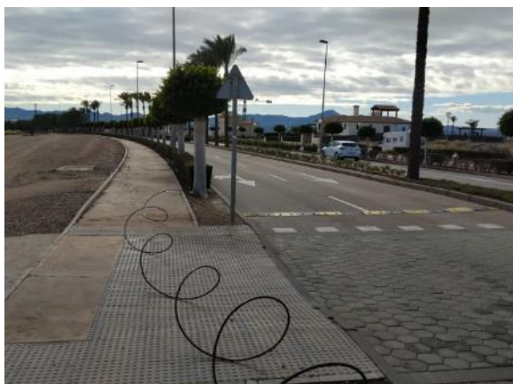
Main Road - From Sales Booth to Black Gravel Round. (870 ml PE Ø16 & 31 links)
