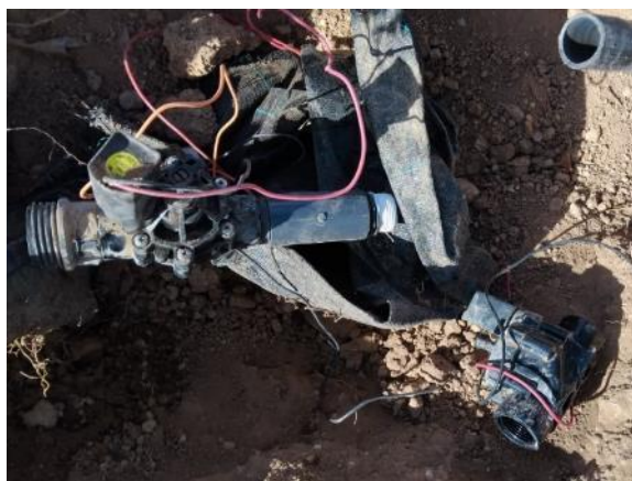
Main Road left near the hotel (change solenoid valve 1")
