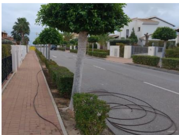
Phase 2 - Belgium St. Num. 21-1 and 40-2 (400 ml PE Ø16 and 6 links)
