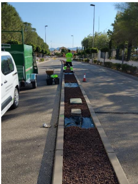
Phase 8 entrance road (irrigation line replacement)
