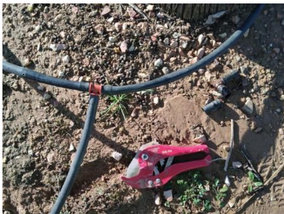
Garden Security (1 ml PE Ø16 and 1 T link)
