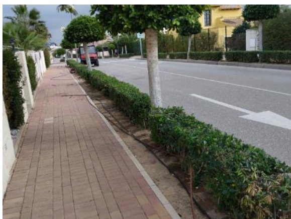
Phase 1 - Austria St. Num. 5-7 (35 ml PE Ø16 and 2 links)
