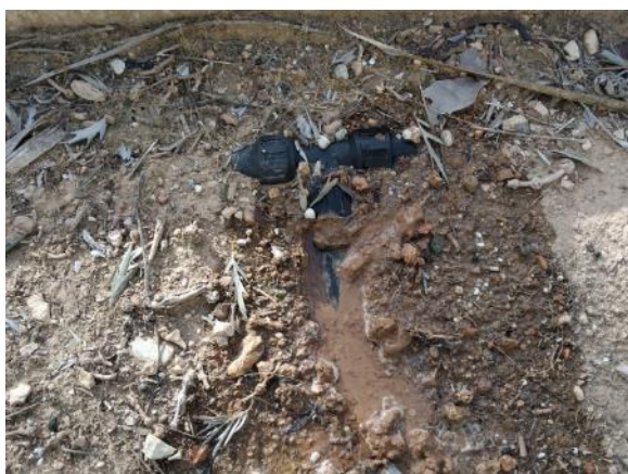
Phase 6 Zone B - Various repairs (4 ml PE Ø16 and 8 links)
