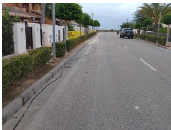
Phase 2 - Belgium St. Num. 21-1 and 40-2 (400 ml PE Ø16 and 6 links)
