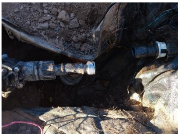
Main Road left near the hotel (change solenoid valve 1")
