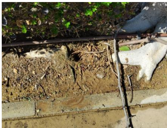
Phase 6 - Front Garden (20 ml PE Ø32 and 2 links)
