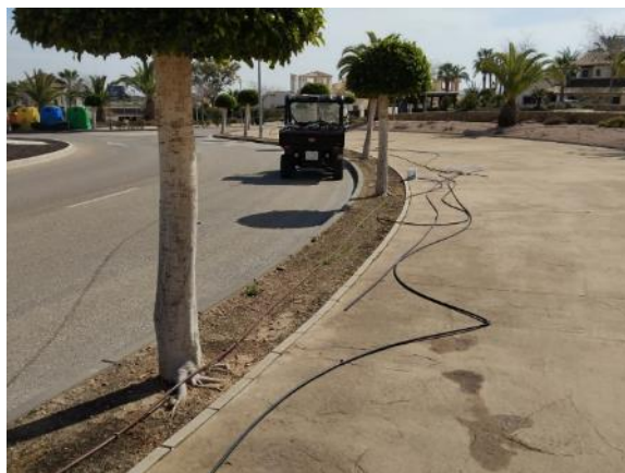
Phase 7 Oasis - Paseo Alameda and Round. (215 ml PE Ø16 and 80 punctured droppers)
