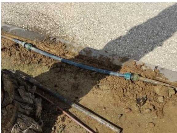
Main Road Median - Next to Storage Area (1.5 ml PE Ø32 and 2 links)
