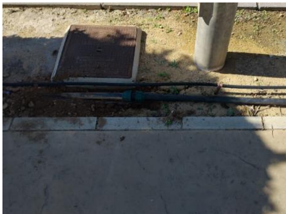
Phase 6 - Front Garden (20 ml PE Ø32 and 2 links)
