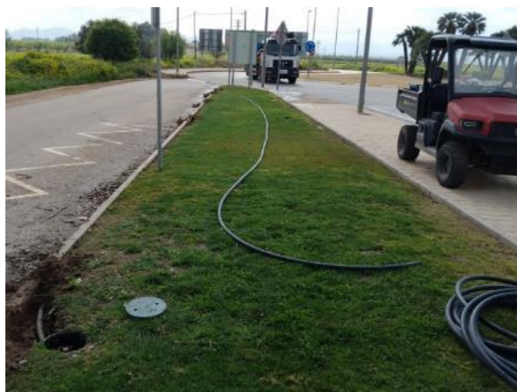
Right entrance - Cypress hedge alignment Totem (60 trees, irrigation setback, 6 diffusers, 30 ml PE Ø32, 1 valve Ø32, 4 links Ø32, 42 ml PE Ø16, 1 Solem 1E programmer, 1 solenoid valve and 1 valve box)
