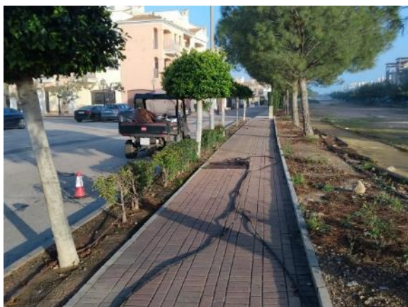
Phase 8 Pueblo Español - Replacement of right drip line (40 ml PE Ø16 and 4 links)
