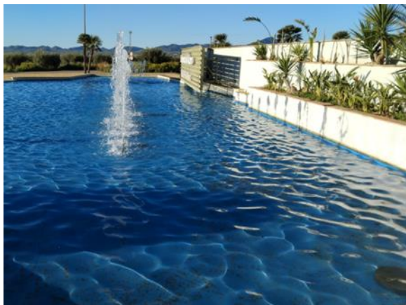
Entrance Fountain - Cleaning leaf accumulation in pump and floating area
