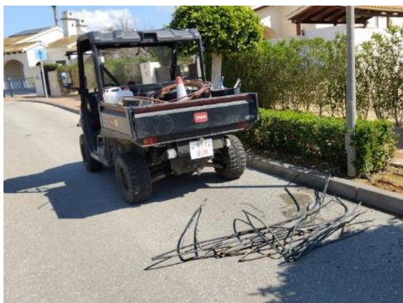
Phase 1 - Replenishment Australia (35 ml PE Ø16, 4 links and 1 Solem 1E programmer)
