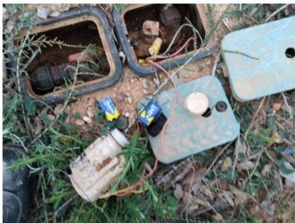
Phase 2 - In front of C/ Brasil, 30 (programmer battery change)
