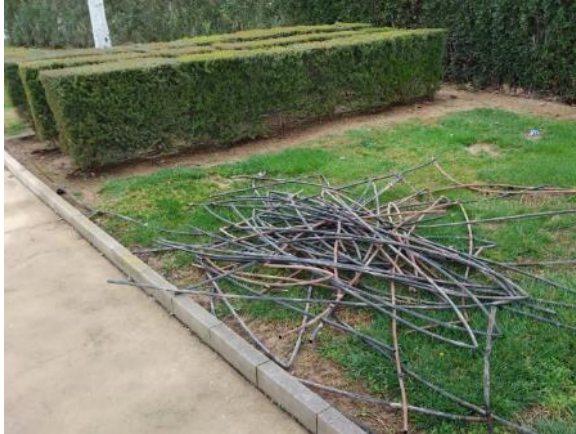
Garden Pictures - Drip line replacement (180 ml PE Ø16, 36 links and 1 Solem 1E programmer)
