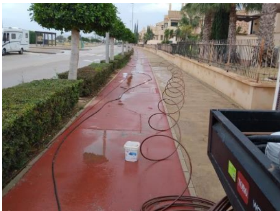
Phase 7 Oasis - Drip line replacement (485 ml PE Ø16, 12 links and 20 droppers)
