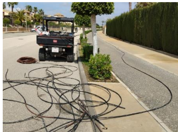
Phase 1 - Replacement in P. Alameda Right (265 ml PE Ø16 and 9 links)
