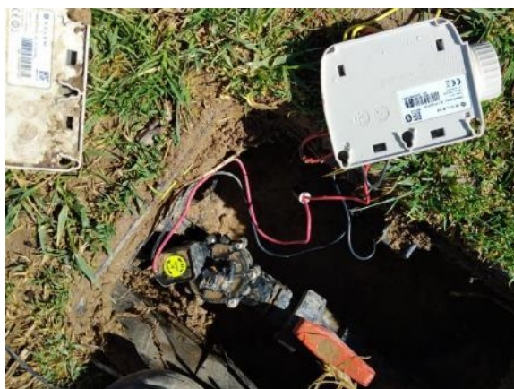
Right entrance - Cypress hedge alignment Totem (60 trees, irrigation setback, 6 diffusers, 30 ml PE Ø32, 1 valve Ø32, 4 links Ø32, 42 ml PE Ø16, 1 Solem 1E programmer, 1 solenoid valve and 1 valve box)
