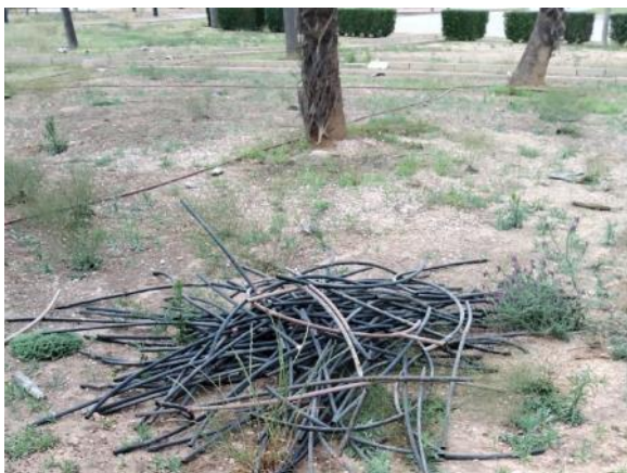
Garden behind the Security Guards - Drip line refill (180 ml PE Ø16, 44 drippers)
