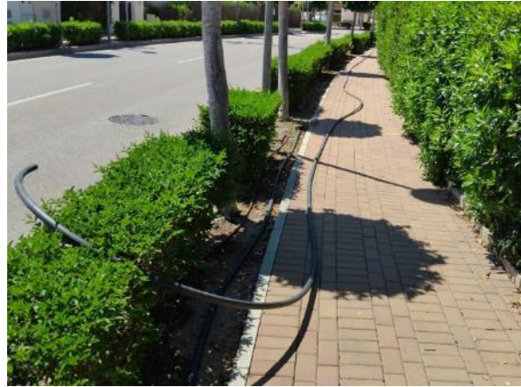
Phase 2 - C/ Belgium 35-33 (replacement 33 ml PE Ø32, 2 links)
