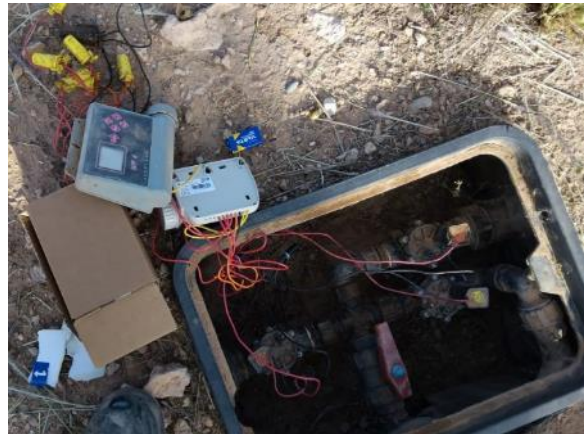
Main road - Flowerbed next to the Clubhouse parking lot (replacement of Rain Bird programmer broken by Solem 4E)
