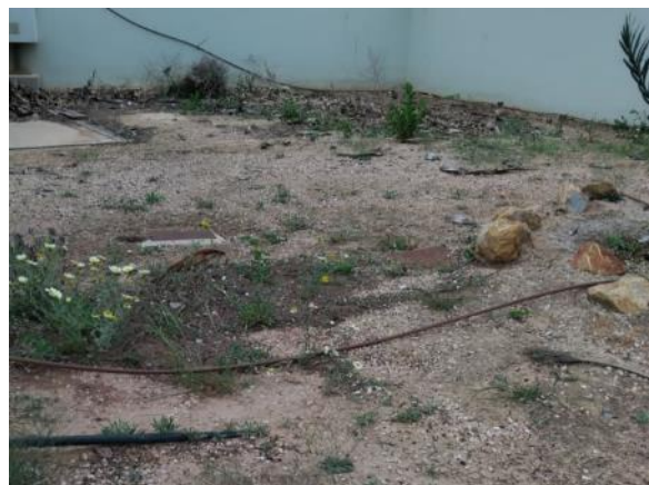
Garden behind the Security Guards - Drip line refill (180 ml PE Ø16, 44 drippers)
