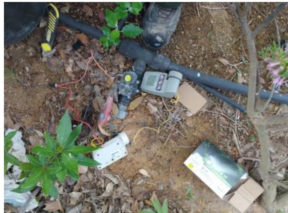
Cuadros Garden (next to Olivos mailboxes) - Rain Bird programmer replaced with Solem 1E
