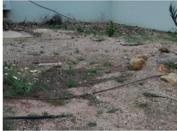
Garden behind the Security Guards - Drip line refill (180 ml PE Ø16, 44 drippers)
