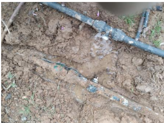
Main vial - Garden Squares (1 solenoid valve 1", 1 ml PE Ø50, 1 T-connector)
