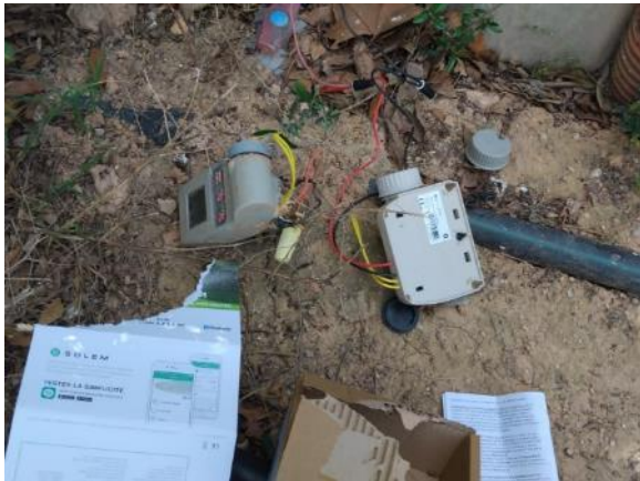
Main road - Guardhouse next to lighting pole (Solem 1E programmer change)
