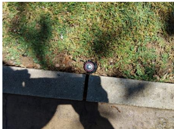
Entrance - Lawn (replacement of 12 sprinkler irrigation nozzles)
