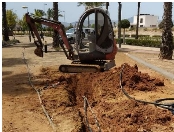
Phase 6 - Olivos A (repair of 10 ml PE Ø32 pipe, 4 links)
