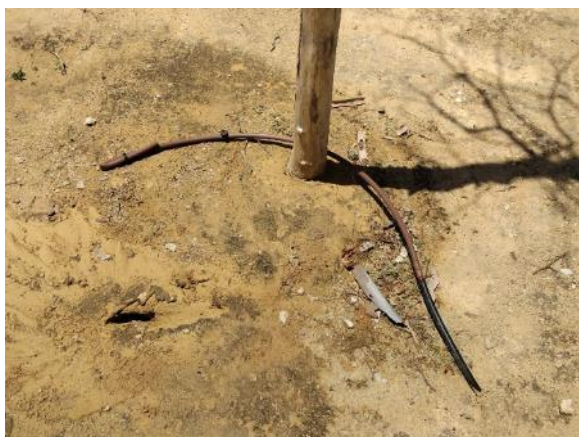
Phase 6 - Olivos Garden B (repair ring 2 ml PE Ø16, 2 links, 2 drippers)
