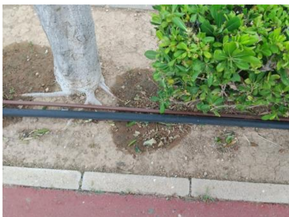
Main Road - C/ Vistas Green garden (refill 70 ml PE Ø16, 6 links)
