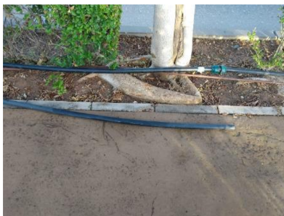
Main Road - Sports fields (2 ml repair PE Ø32, 2 links)
