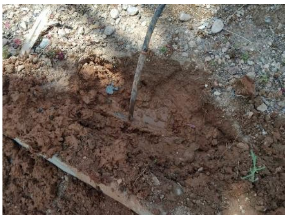
Phase 6 - C/ Guinea garden (repair leak 0.5 ml PE Ø16, 2 links)
