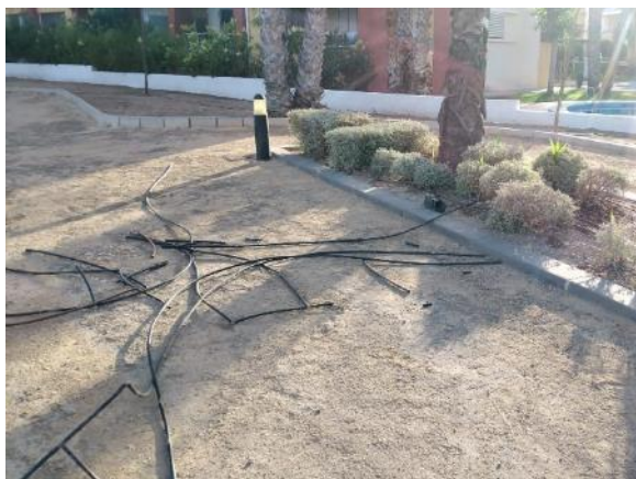
Phase 6 - Olivos A (repair of old cracked pipe 23 ml PE Ø16, 6 links)
