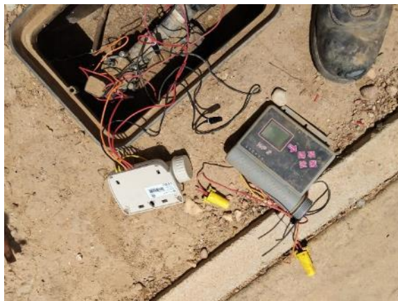
Main Road Right - Maintenance (replacement of Rain Bird programmer with a new SOLEM)
