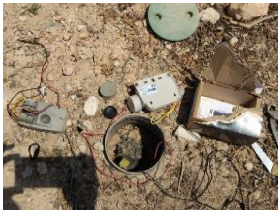
F1 Roundabout - EUM (replacement of 1 Solem 1E programmer, valve box and junction)
