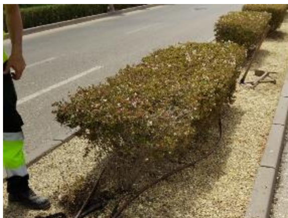
Main Road (median) - from guardhouse to Olivos (replacement of 70 ml PE pipe Ø32 and 2 links)
