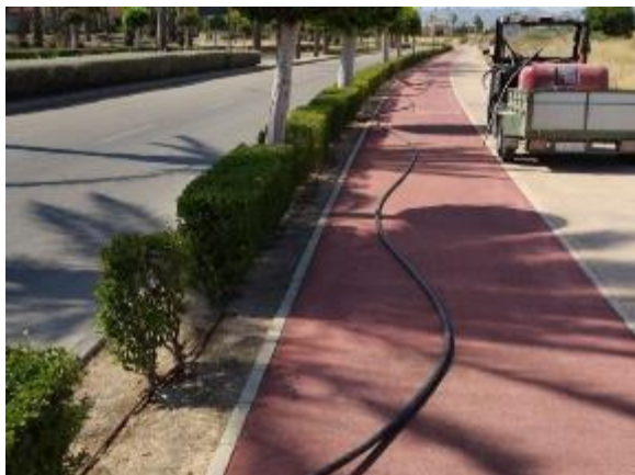
Main Left Road - Opposite Olivos A (repair of old cracked pipe 40 ml PE Ø32, 2 links)
