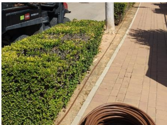
Phase 2 - C/ Bahamas 34 to 48 (replacement of 90 ml PE Ø16 pipe, 7 links)
