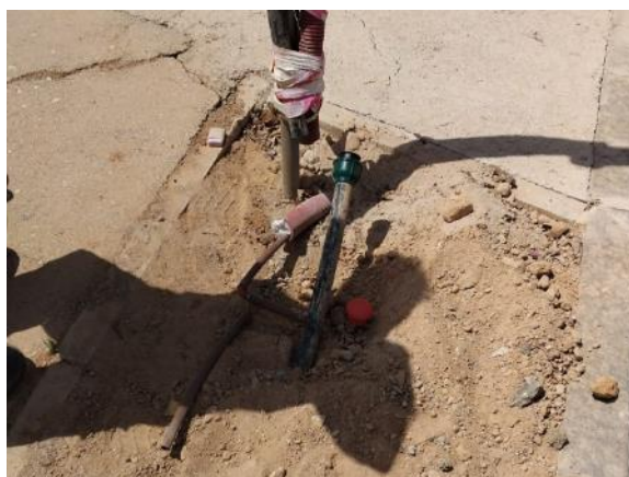
Phase 7 Oasis - Transition to New Housing (installation of 2 plugs Ø32, 12 ml PE pipe Ø16, 2 connectors)
