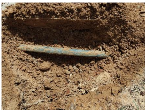
Phase 6 - Back Garden (repair of 1 ml PE Ø32 pipe, 2 links)
