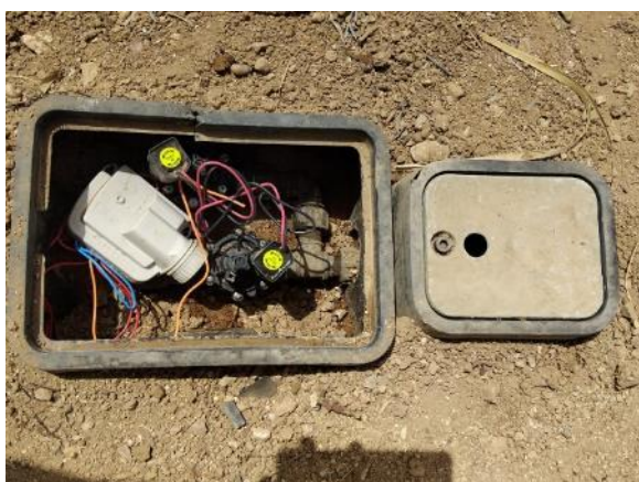
Phase 6 - Olivos B (replacement of 1 Solem 2E programmer and 2 1" solenoid valves)
