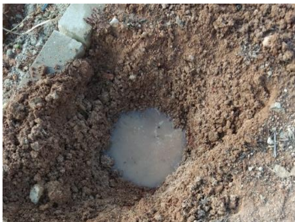
Phase 6 - Back Garden (replacement of old pipe 70 ml PE Ø32, 2 links)
