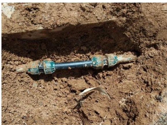
Phase 6 - Back Garden (repair of 1 ml PE Ø32 pipe, 2 links)
