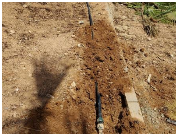
Phase 6 - Back Garden (replacement of old pipe 70 ml PE Ø32, 2 links)
