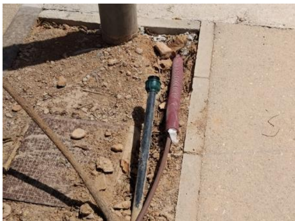
Phase 7 Oasis - Transition to New Housing (installation of 2 plugs Ø32, 12 ml PE pipe Ø16, 2 connectors)
