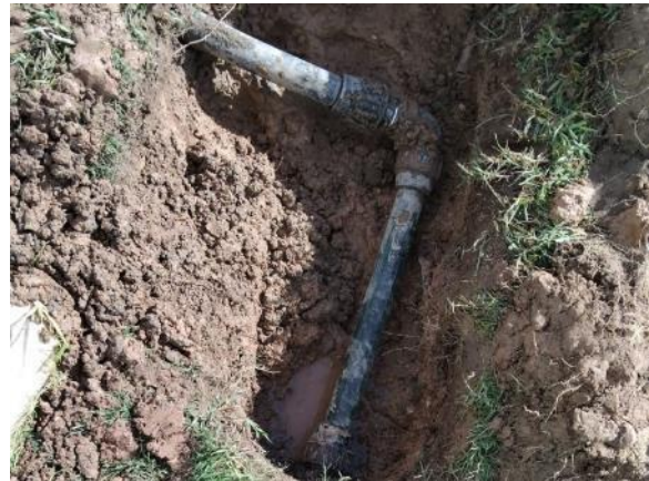
Entrance - Roundabout (repair 0.5 ml PE Ø50, 1 elbow)
