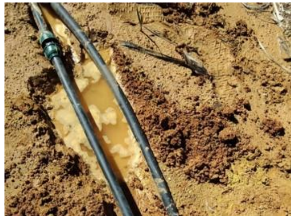
Phase 6 - Olivos A (repair 0.5 m of PE Ø32; 2 links)
