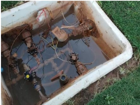
Entrance - Roundabout (repair 0.5 ml PE Ø50, 1 elbow)
