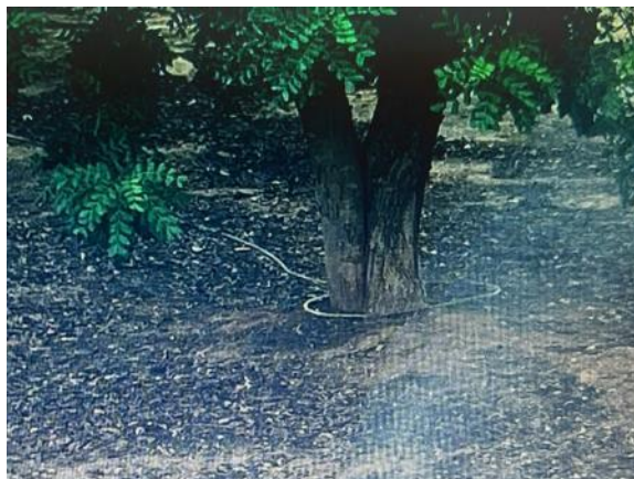
Phase 6 - Guinea St., Algarrobos garden (repair of 2 lm of Ø32 PE, 2 links)
