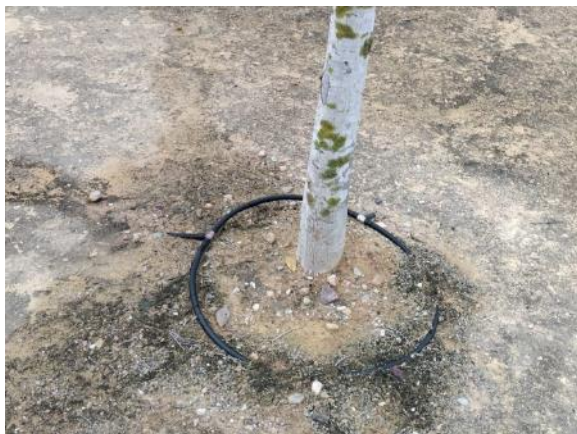
Bélgica Ave. - Left side of entrance (repair of 0.5 m of PE, Ø16, 1 link)
