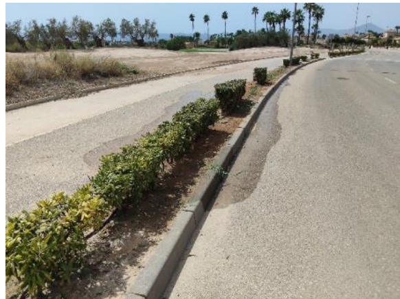
Phase 1 - Road B (repair 1 ml Ø16 PE, 2 links)
