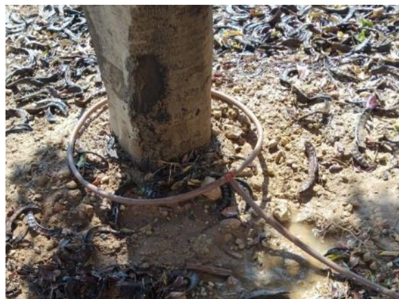
Phase 6 - C/ Guinea (repair 1 ml PE Ø16, 1 T link)
