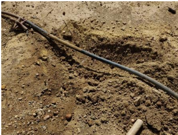
Phase 6 - C/ Guinea (repair 0.5 ml PE Ø16, 2 links)
