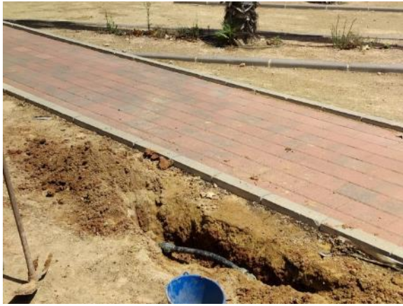
Phase 6 - Olivos B Garden (repair of 1 ml Ø32 PE pipe, 2 links)
