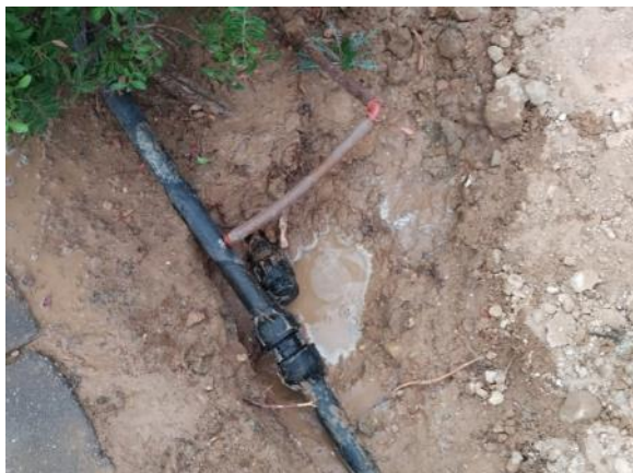
Phase 7 - Oasis (repair 1 ml PE Ø32, 1 link, and 2 caps)
