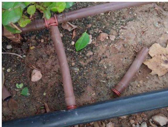
Main Road (right) - Opposite football field (repair 0.5 ml PE Ø16, 1 link)
